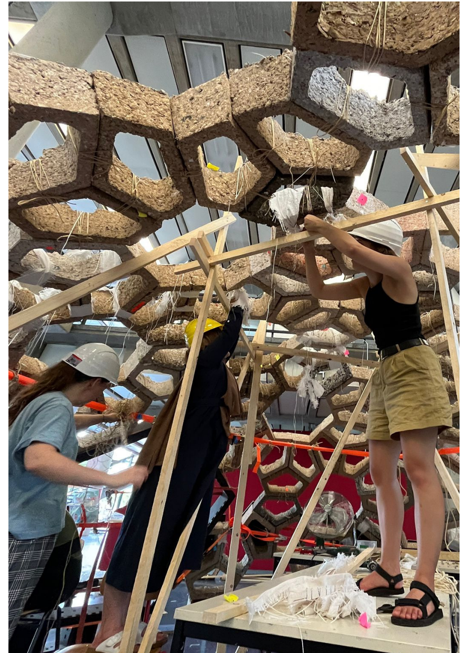
Students building the Crush Up pavilion. July 2022.
